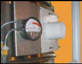
Pressure indicator measures the filter resistance
