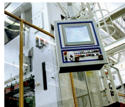
— Retrofitting on a press
