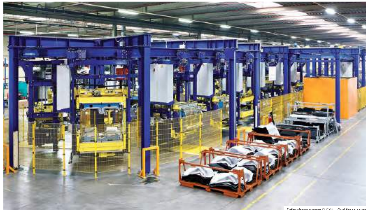
Safety fence system FLEX II – Oval fence course
